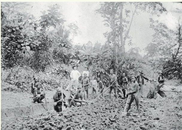
Pembangunan jalan di Nias Selatan Construction of a road, South Nias
